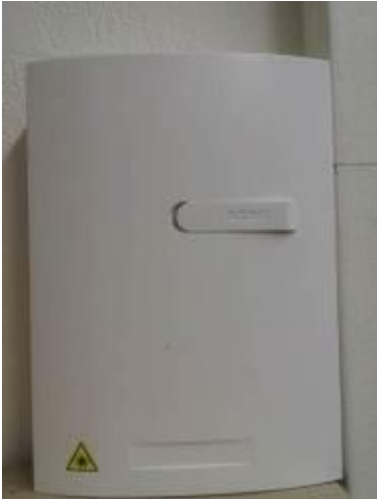
Figure 11 : PBO ACOME mono fibre
